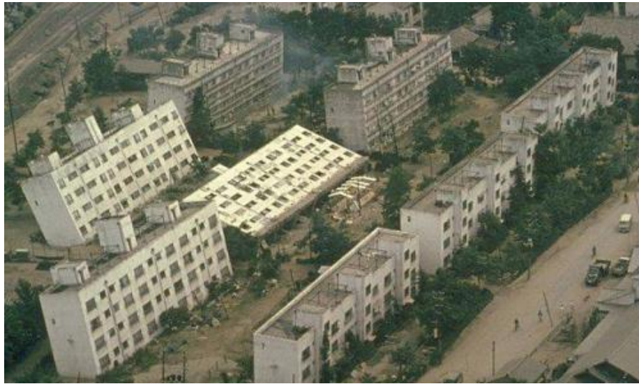
Figure 3-18: Loss of Bearing Capacity due to Soil Liquefaction from Niigata, Japan 1964 Earthquake (Niigata Earthquake, 1964).
